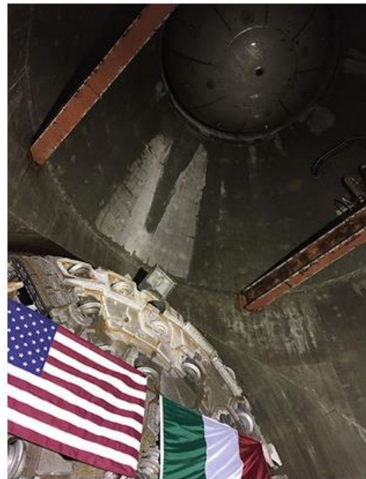
TBM breakthrough into precast concrete intake structure – the circular plug at the top is holding back Lake Mead above
