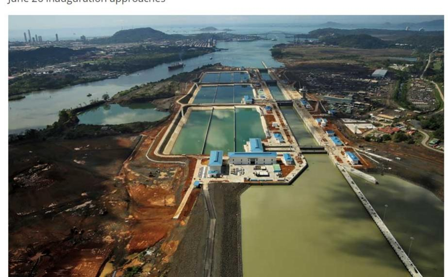
**Sprint to Finish** On the Panama Canal's Pacific Ocean side, crews constructed new locks and water-retention basins and excavated 6.1 km of new canal as part of the third-lane project. *Photo courtesy of Salini Impregilo*
