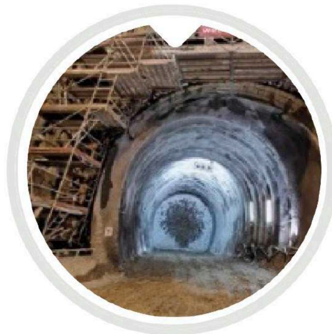
Artificial Ground Freezing
