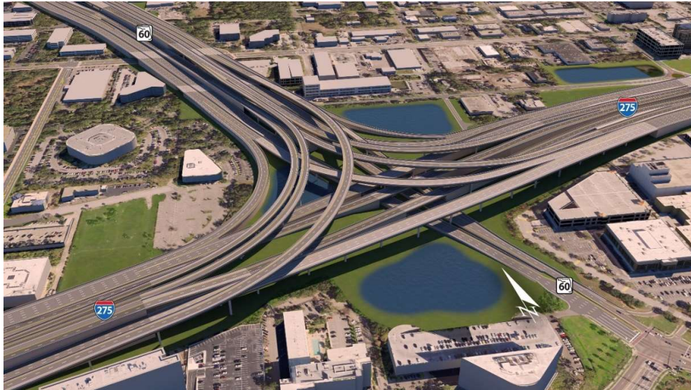
Photo courtesy by Florida Department of Transportation
