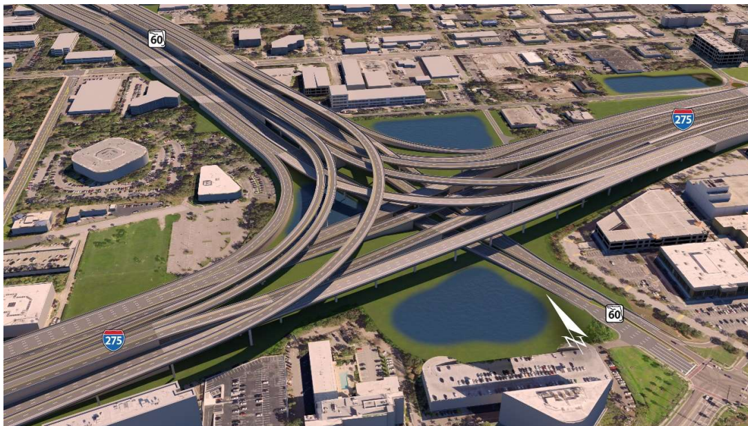
Photo courtesy by Florida Department of Transportation
