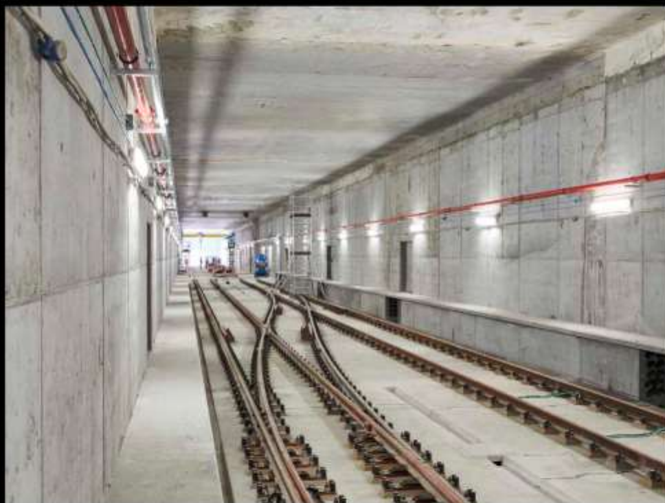
05 of 07 Newly laid track in Milan
