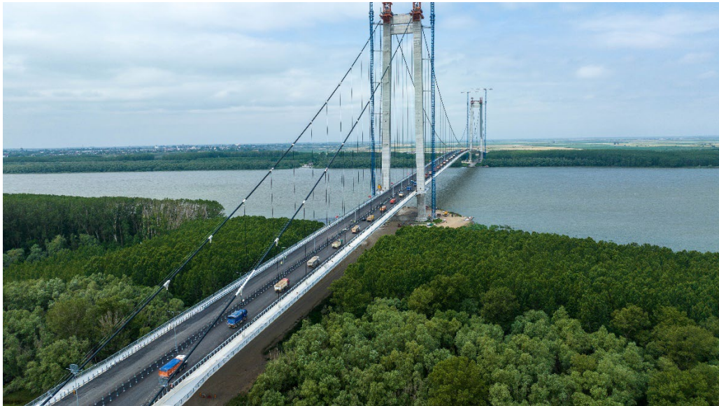
Braila Bridge – Webuild Image Library
