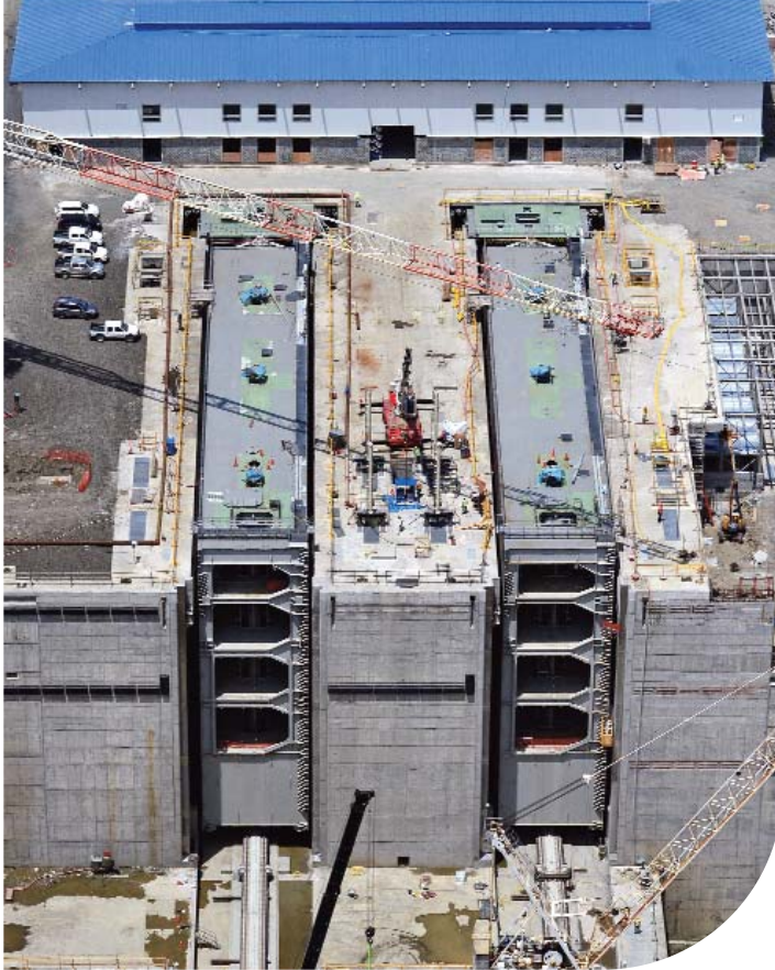
Final stages of gate installation.
