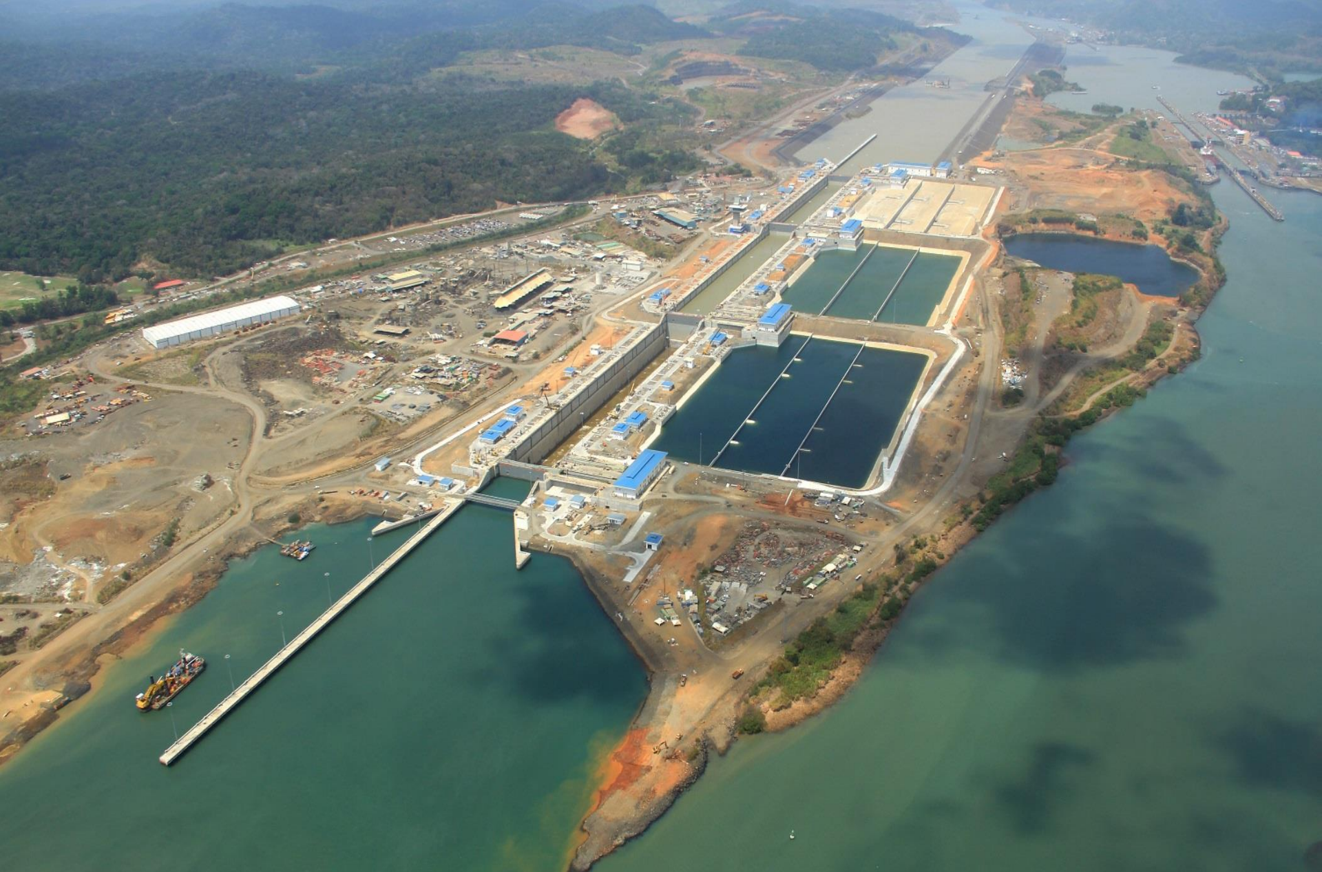
Extension of the Panama Canal – Third set of locks Completion Progress: 95%
