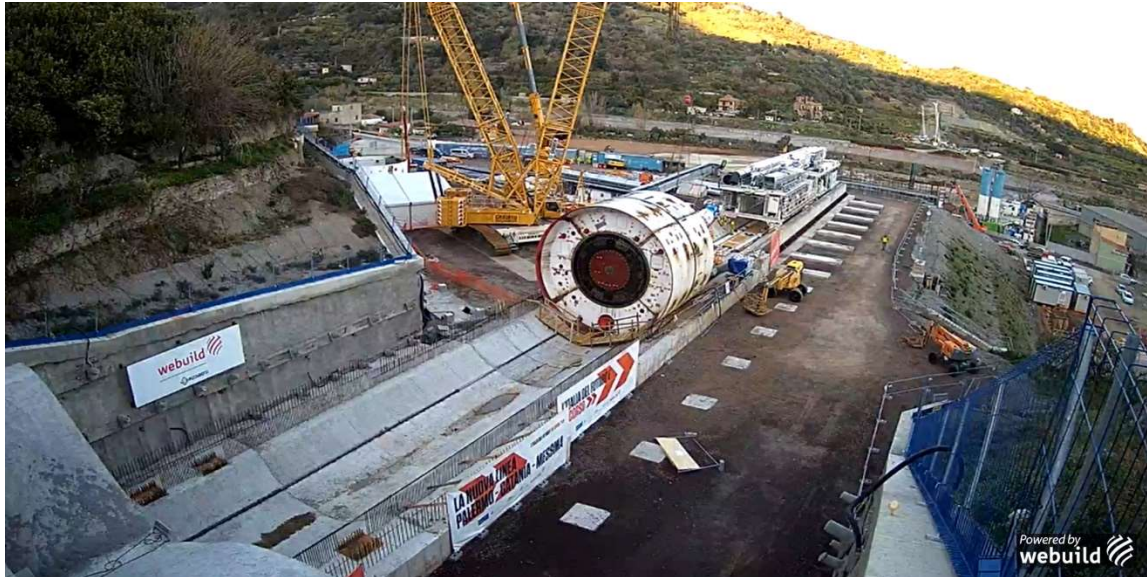
Taormina-Giampilieri High-Speed Railway line section, Sciglio Construction site
