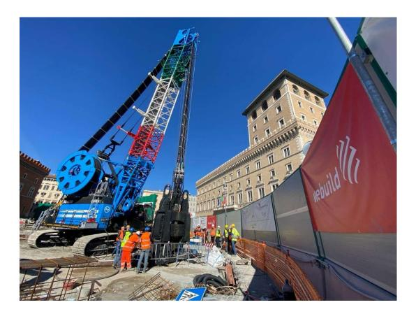
*Rome, February 15, 2024* –During these days the hydro-milling machine, specifically built to excavate the perimeter walls of the new museum station of Piazza Venezia, up to at a record depth of 85 metres has started to function. The station will be a central hub of the Metro Line C, the capital's first self-driving line, commissioned by Roma Metropolitane and built by the consortium company Metro C S.c.p.a., led by Webuild and Vianini Lavori.
