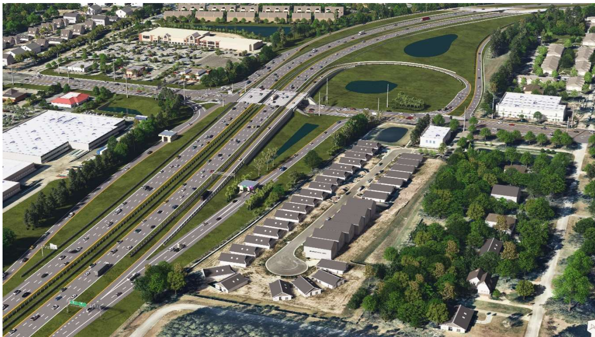
Seminole Expressway / SR417 project – render image
