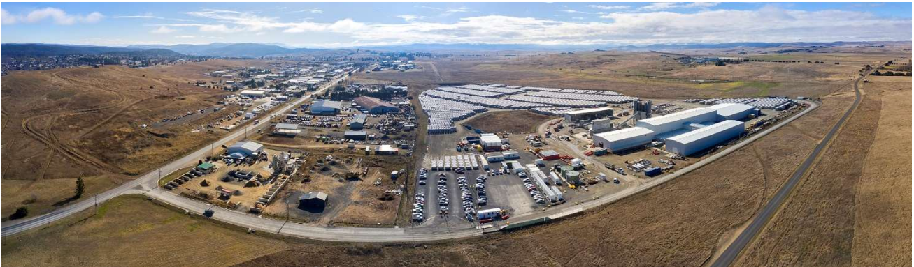
Precast Concrete Segment Factory, Cooma – Credits: Snowy Hydro Ltd.
