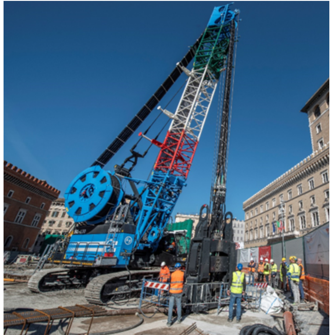
Launch of the TBM - Mechanical mole for excavating tunnels
