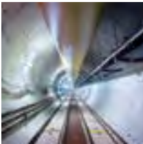
EMIRATI ARABI Abu Dhabi Deep Sewer Tunnel
