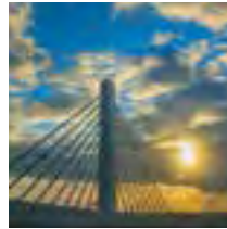
AUSTRALIA Sydney Metro Northwest
