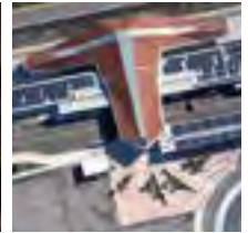
AUSTRALIA Forrestfield Airport Link Perth
