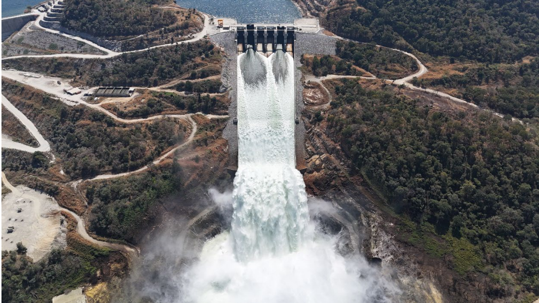
GERD Project ©Webuild Image Library
