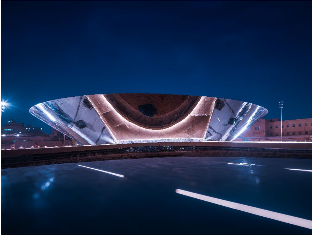
Qasr Al Hokm Downtown Station © Royal Commission for Riyadh City (RCRC)
