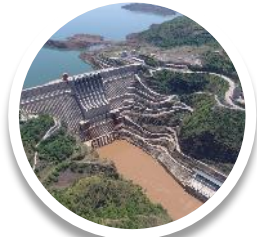
GIBE III HYDROPOWER PROJECT - ETHIOPIA
