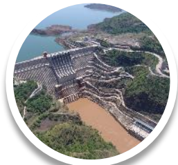
GIBE III HYDROPOWER PROJECT - ETHIOPIA
