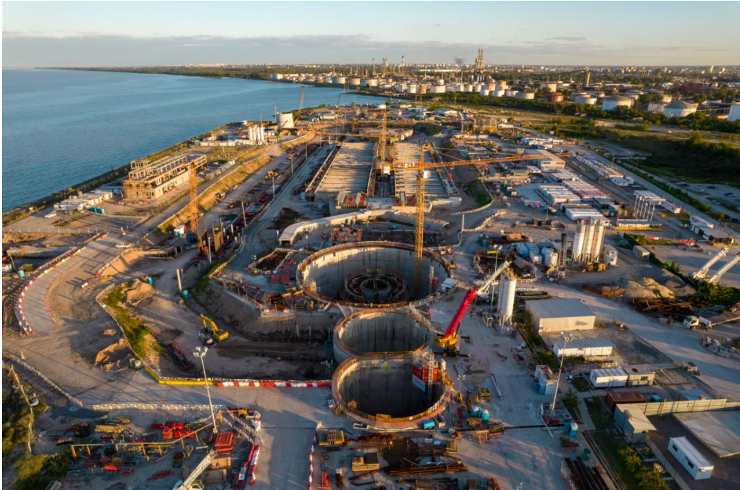
Riachuelo environmental restoration system, Argentina ©Webuild Image Library
