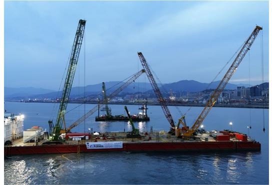
*The material from demolishing the old breakwater is going to be almost entirely used*
