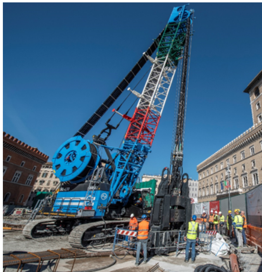
Hydromill at work to create the diaphragms
