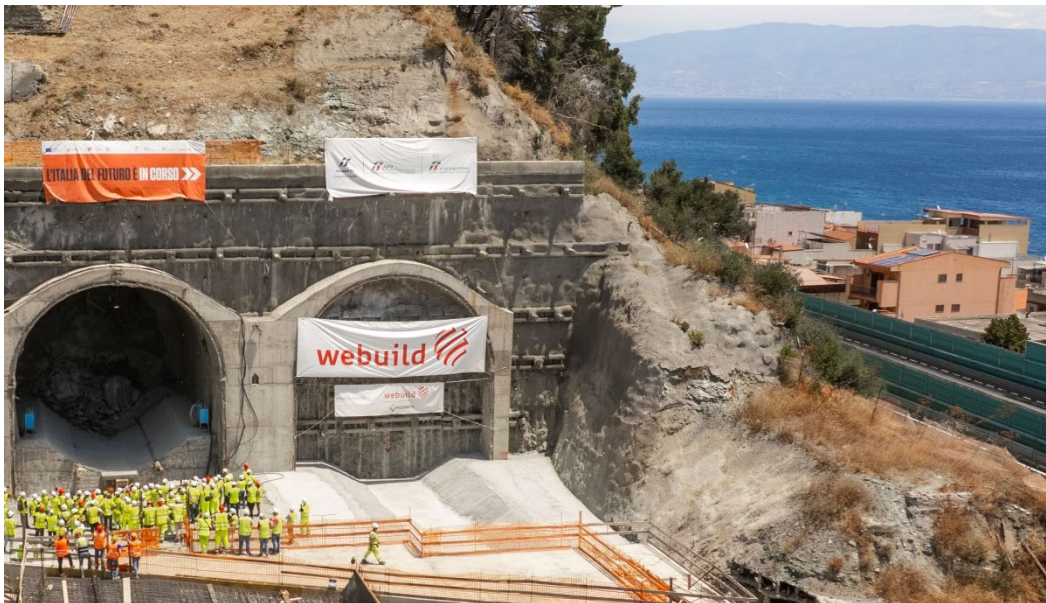
Credits: Webuild Image Library
