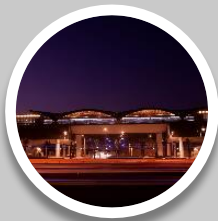
Riyadh Metro Line 3 Saudi Arabia
